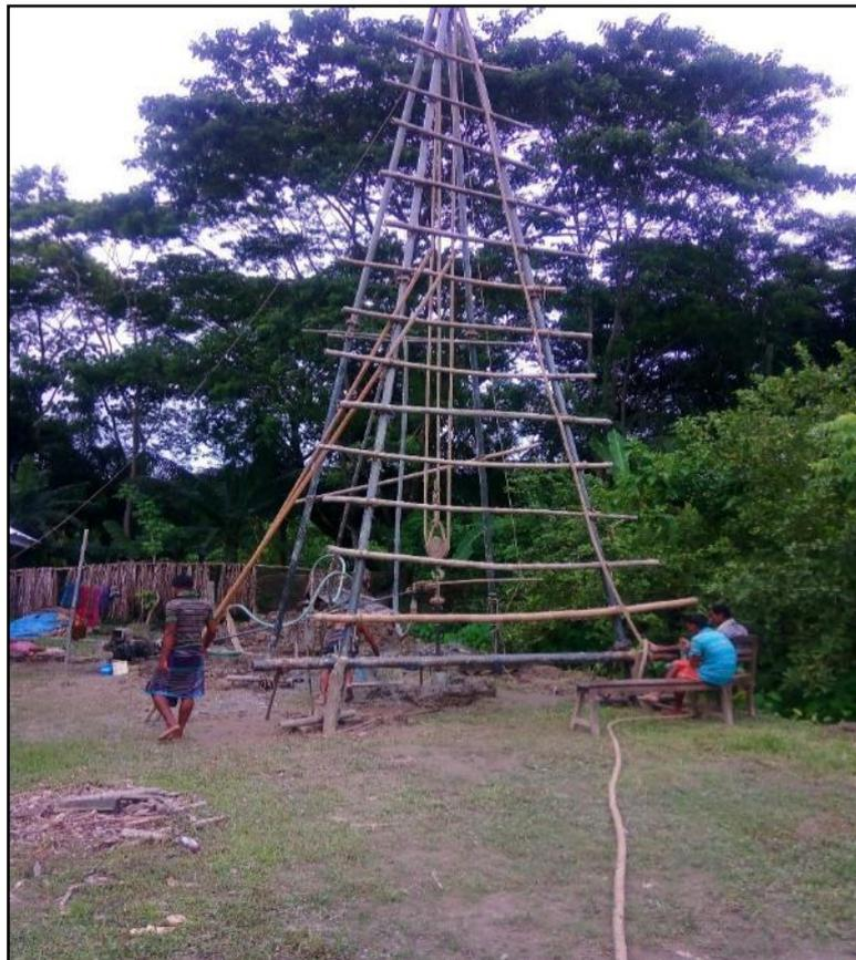
Figure 3: Drilling Procedure of Monitoring well.
