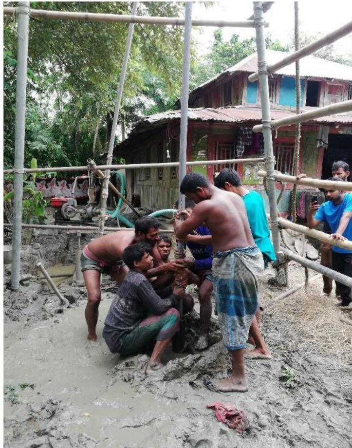
Figure 4: Installation of Monitoring Well
