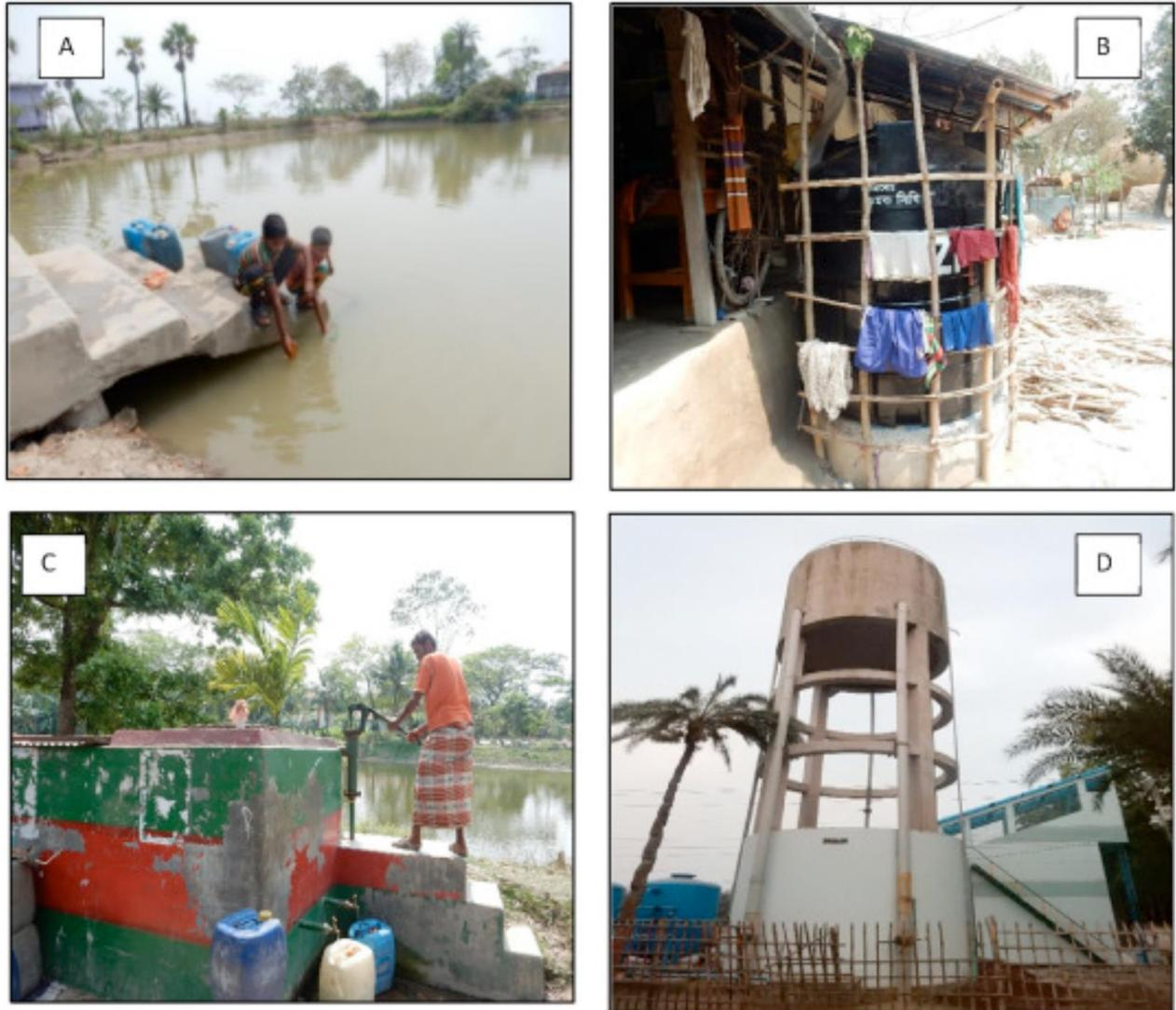
Figure.2. Different drinking water sources in the study areas (A: Collection of pond water for drinking; B: Plastic container for rainwater harvesting; C: Pond Sand Filter (PSF); D: Deep tube well with the overhead tank for water treatment).
