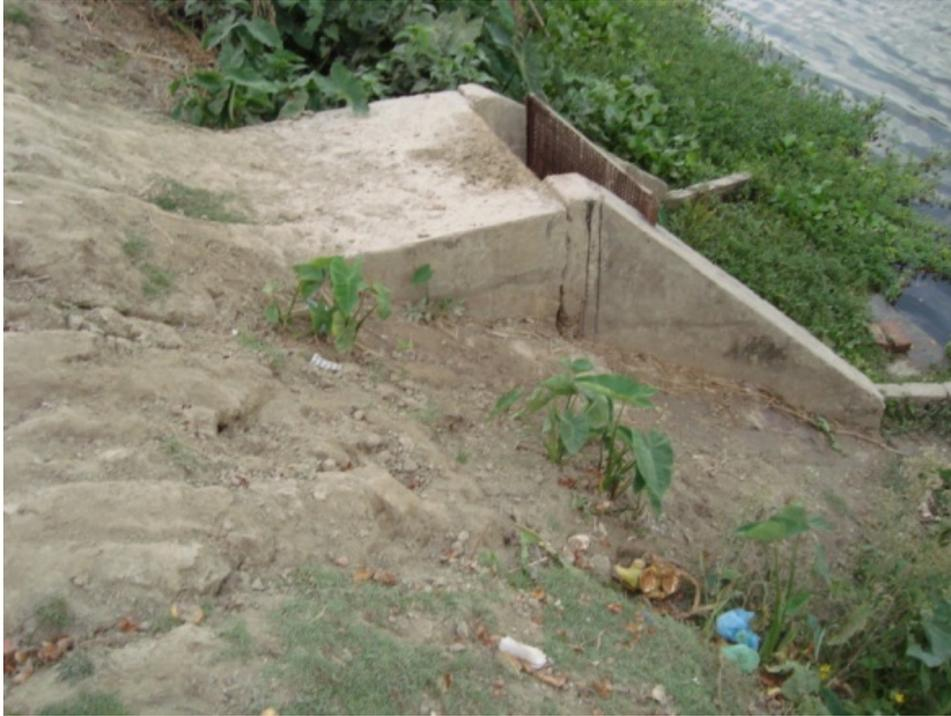
Photograph 2.4: Existing culvert on-road cum bundh through the large water body at Amtali Pourashava.
